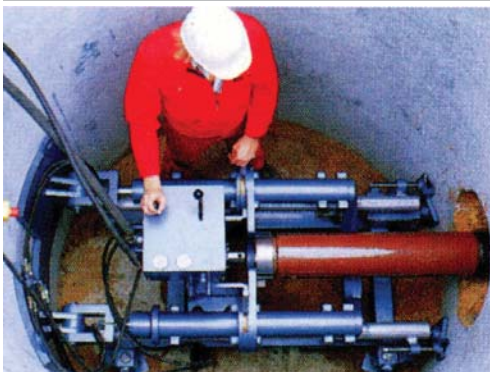
Phase 2 - Augering and removal of soil and the installation of product pipes by microtunneling.
