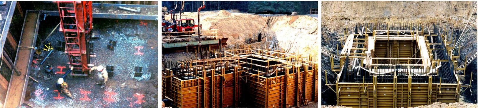
Construction of deep pump stations often requires special construction techniques such as the need for sheet piling, bracing, dewatering, rock removal, sloping, mud mats, and seal courses.
